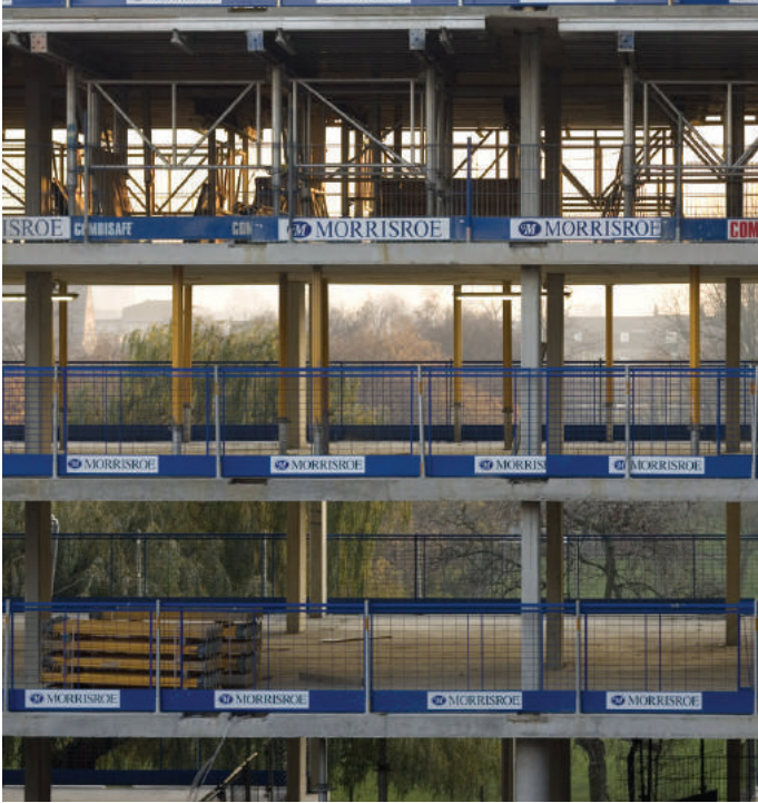
3.10 Frame construction Dec 2006
