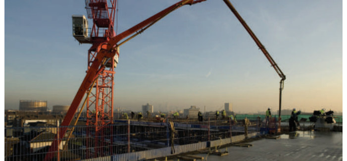
3.11 Roof being poured Jan 2006
