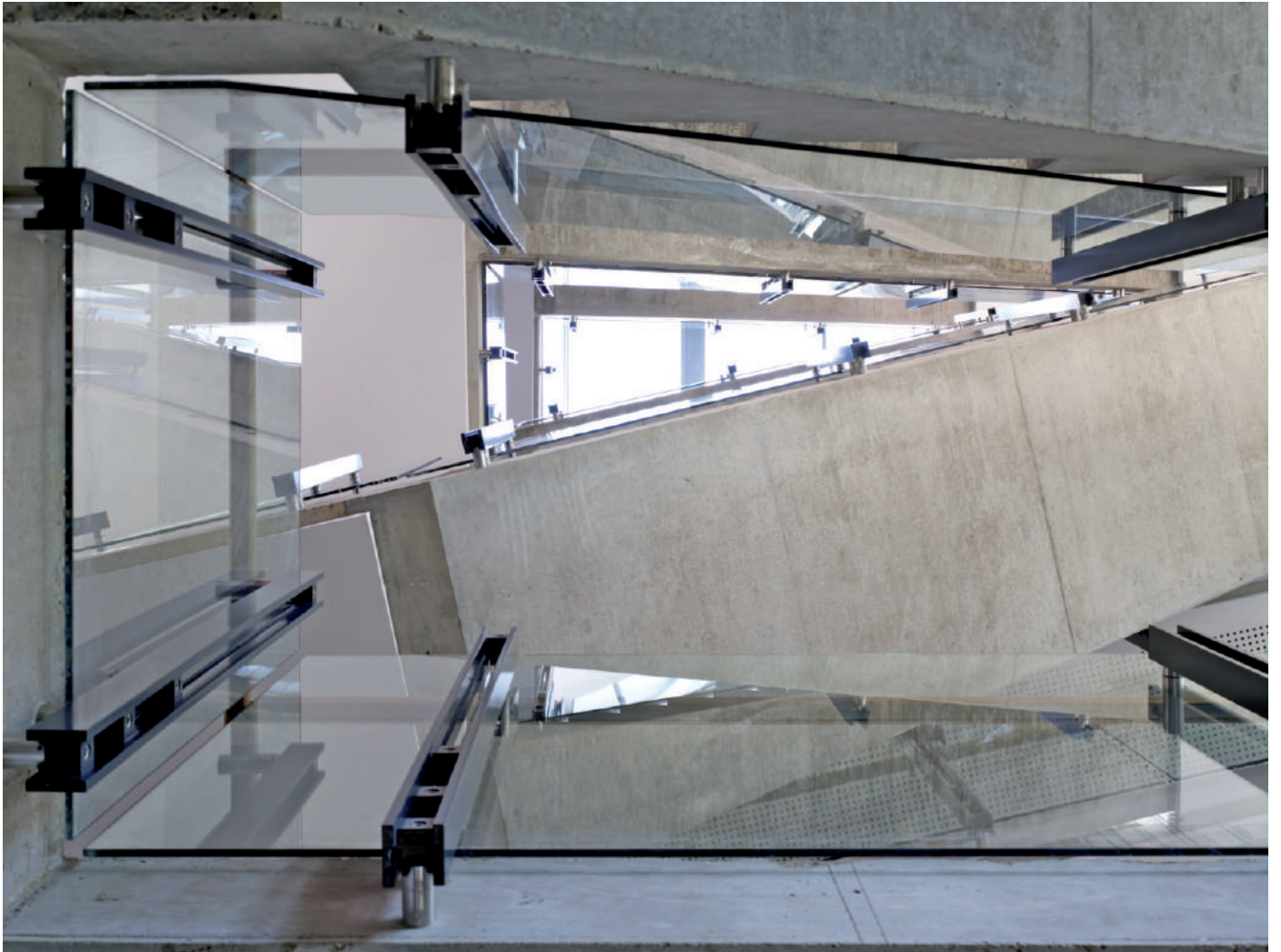
Looking up the main stairwell at the staggered concrete flights
