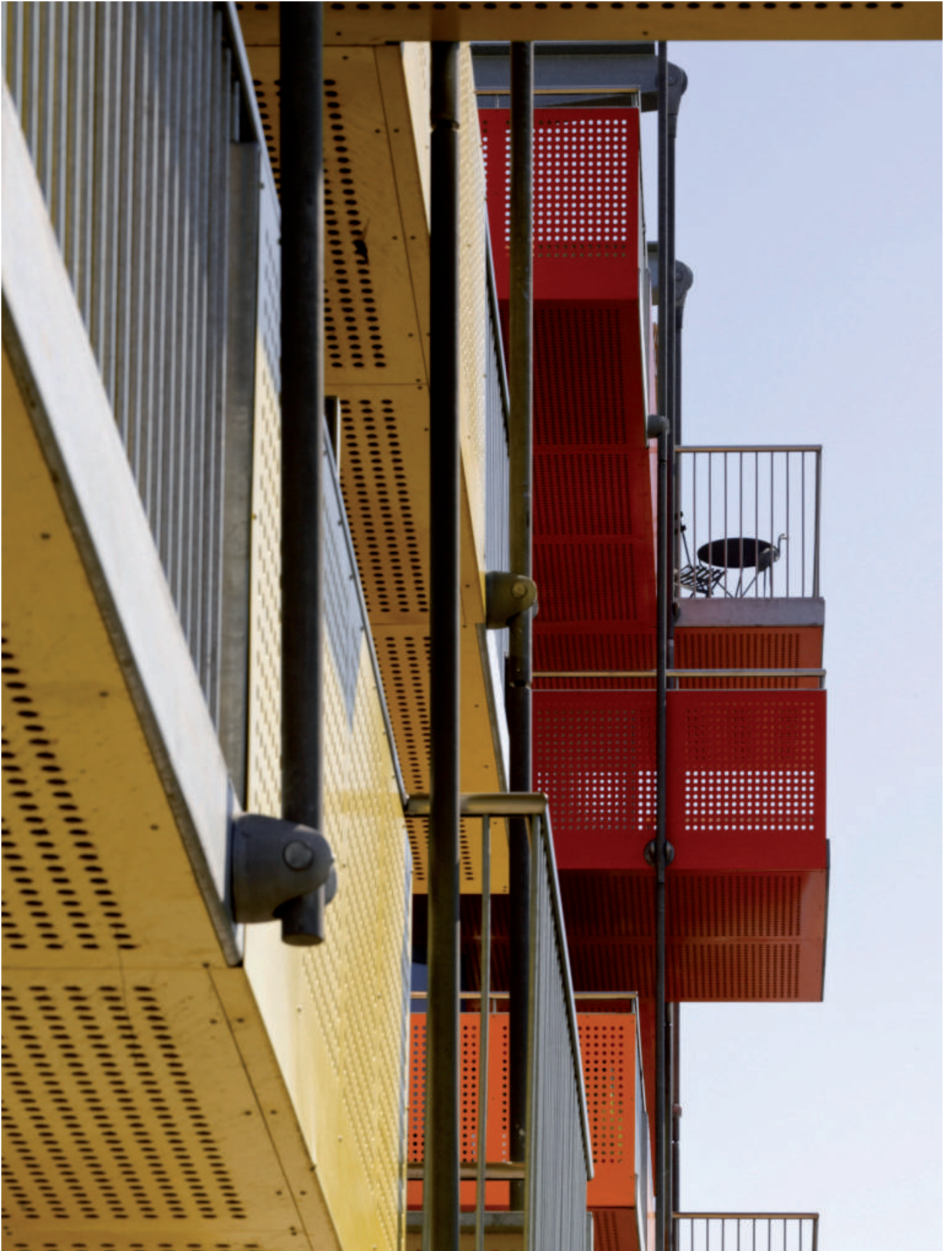
Balconies suspensions rods and bosses
