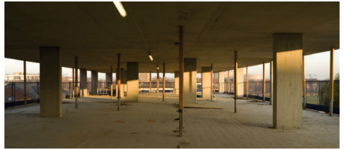
3.12 Flat slabs & balde columns
