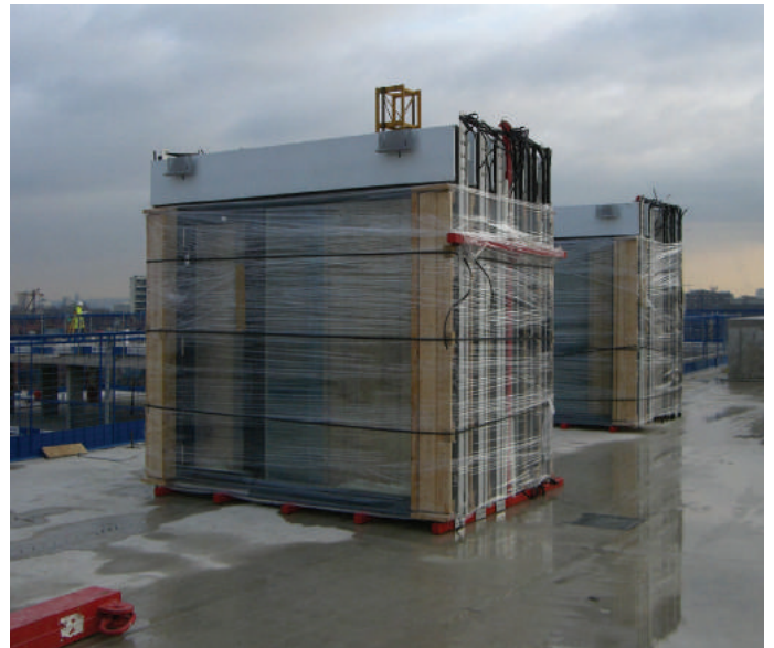
3.14 Unitised cladding panels delivered Jan 2007,
