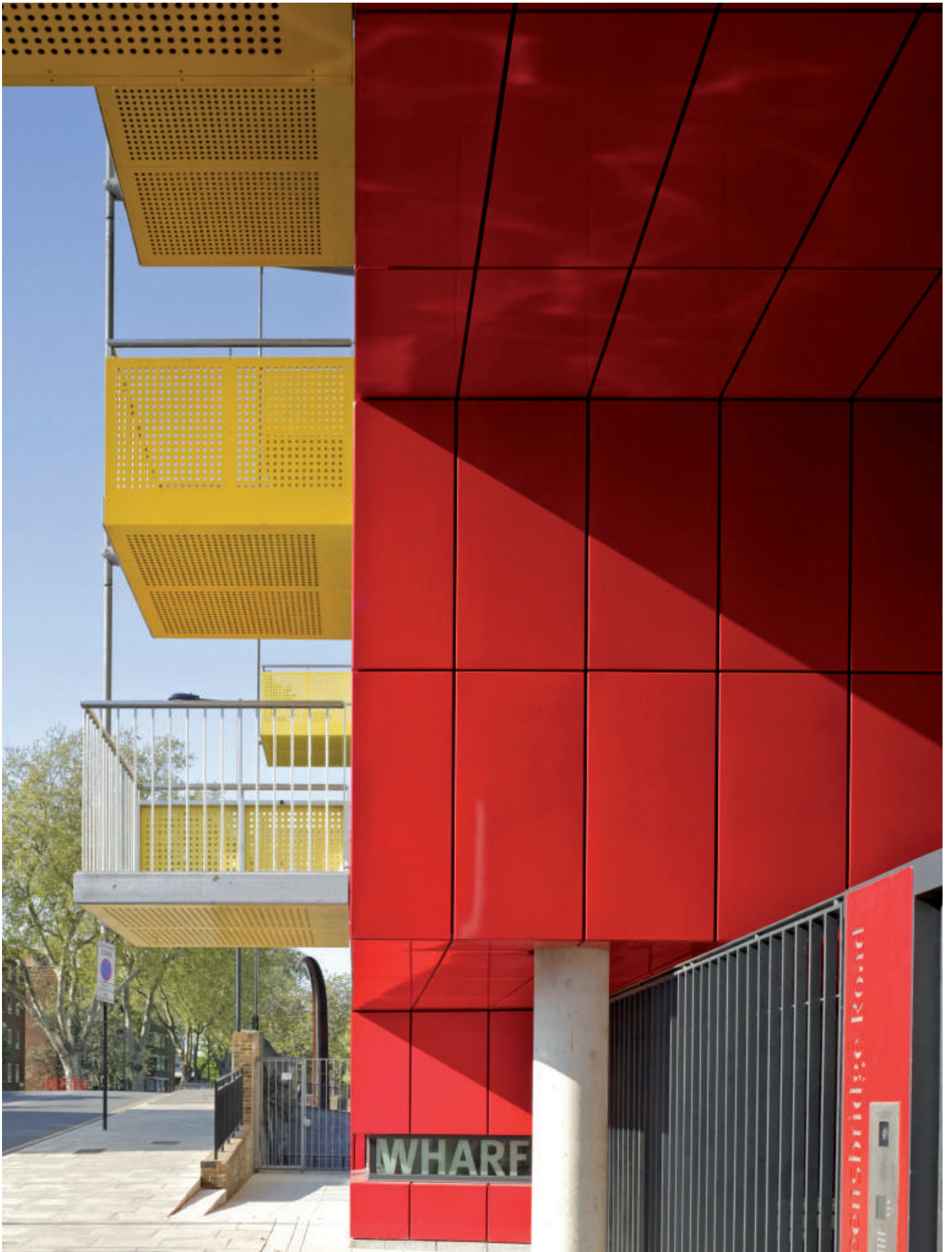
Vitreous enamel cladding at main entrance
