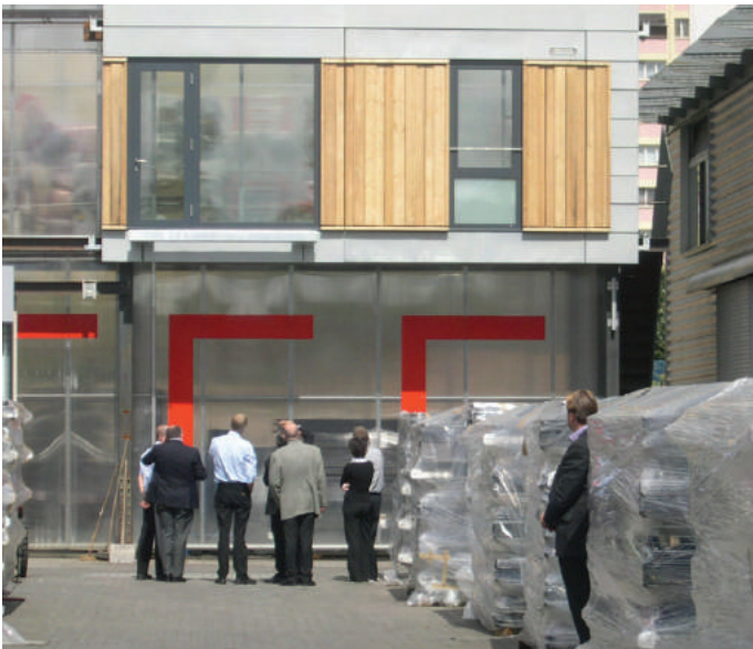
3.13 Cladding proof type inspection July 2006
