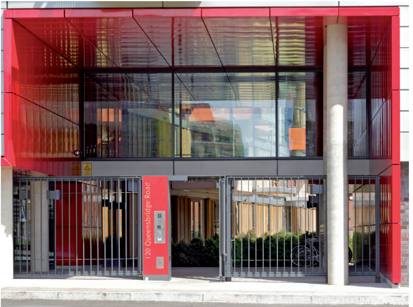
Main enamel lined on Queensbridge Road
