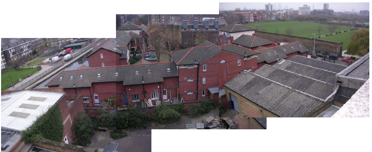
Adjacent view of Gloucester Square roofscape from Adelaide Wharf
