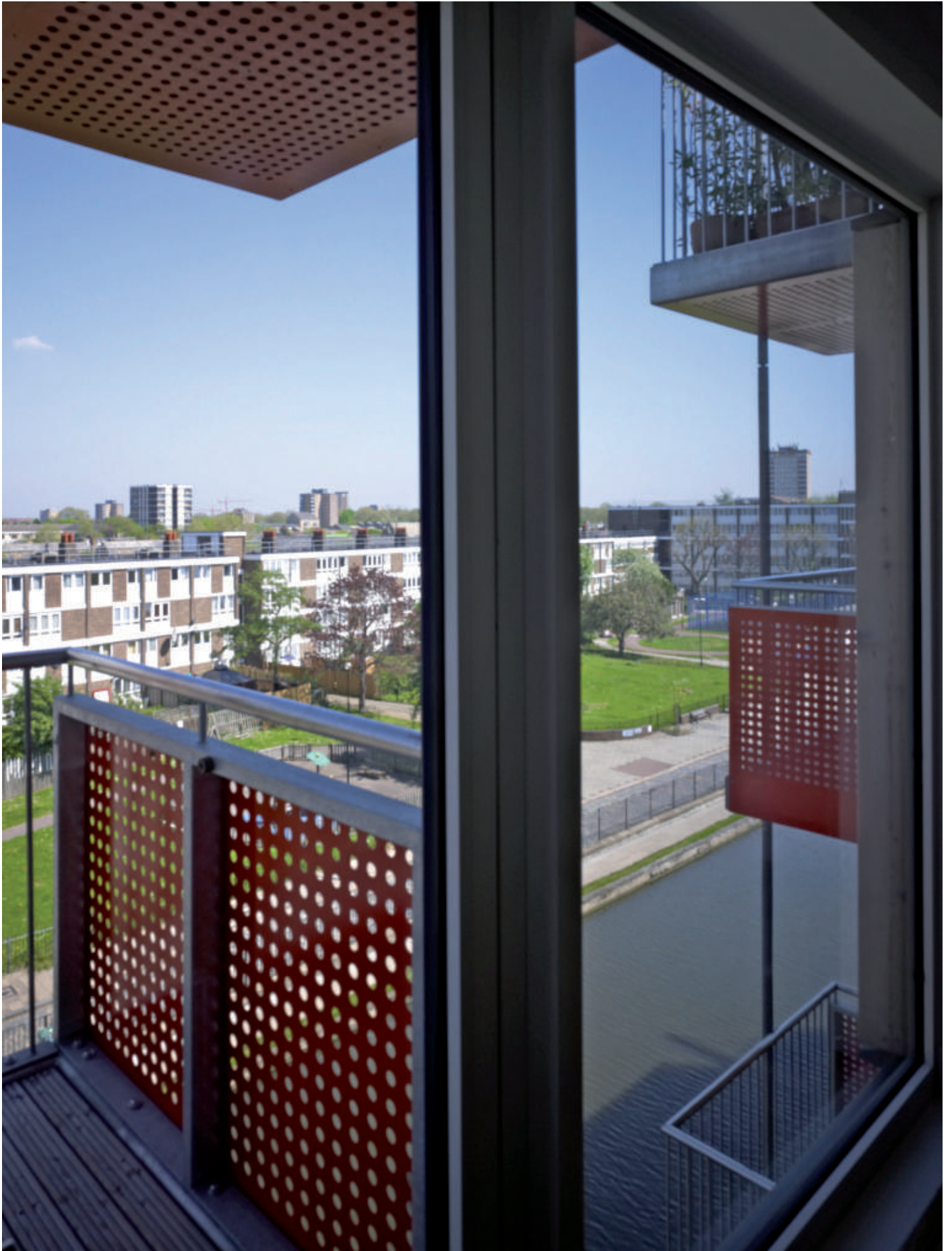
Staggered balconies allow more daylight into the living rooms below
