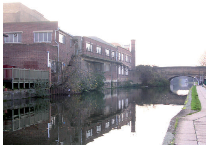
View of canal boundary towards bridge
