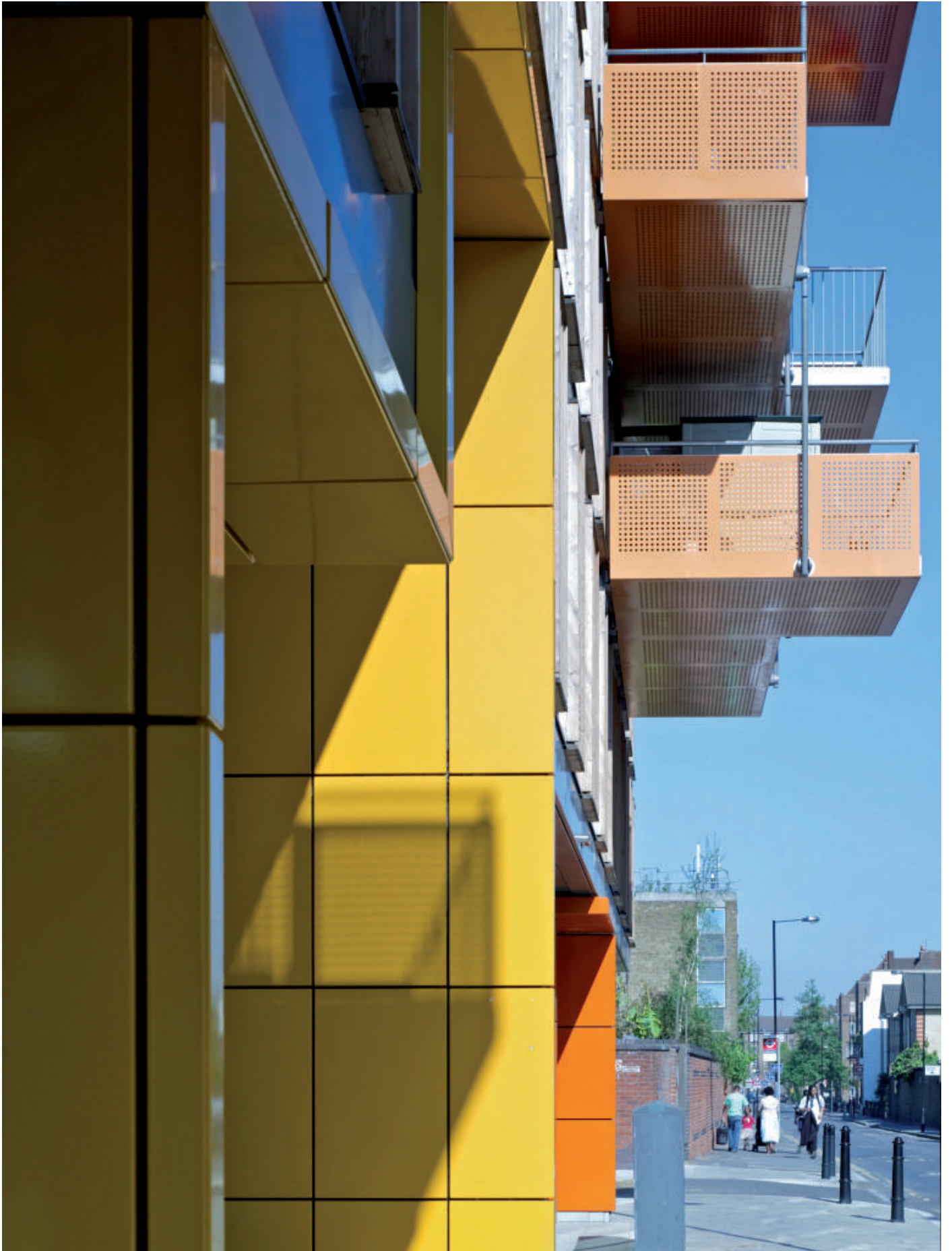
Balconies along Queensbridge Road
