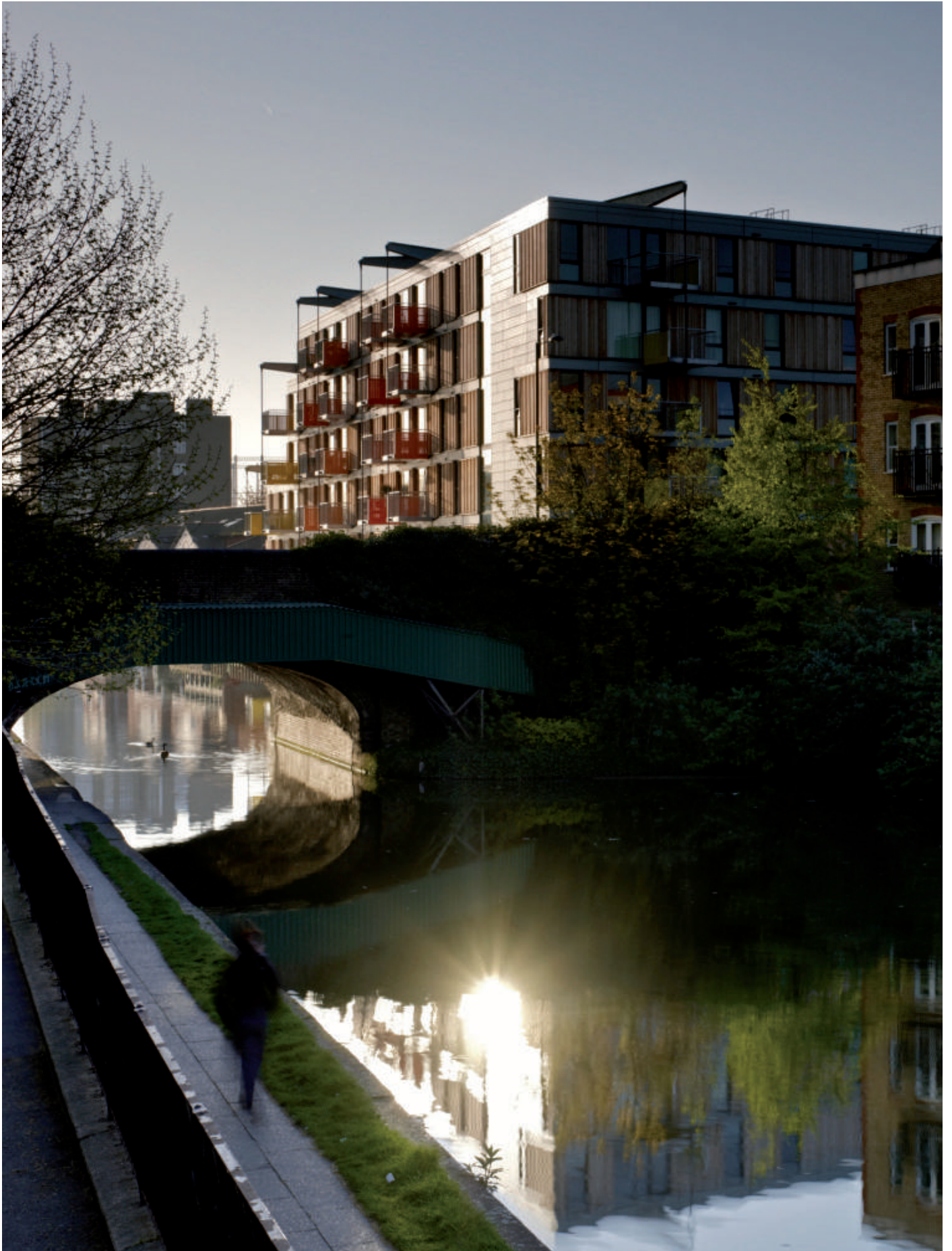
Looking east along Regent's Canal towards Adelaide Wharf
